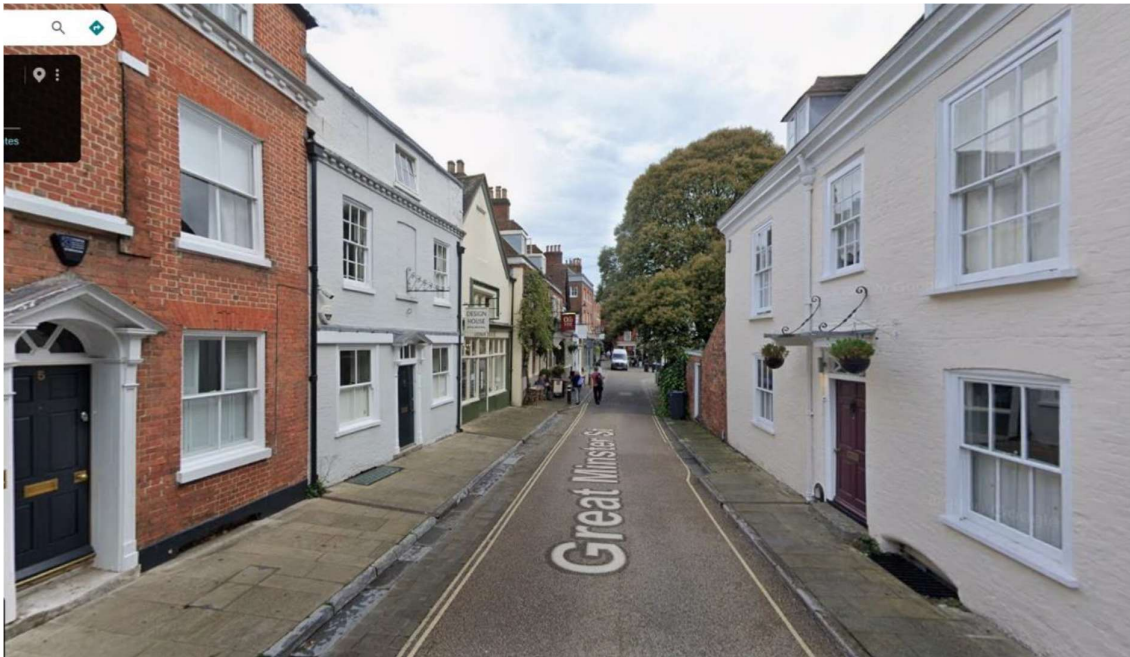
Great Minster Street looking north towards the High Street
